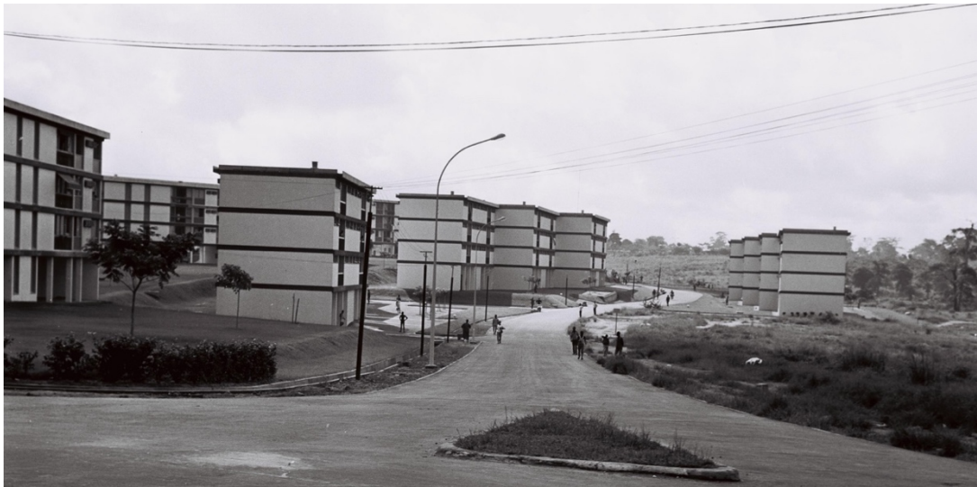
Modern suburb of Abidjan (Ivory Coast) built by local workers under supervision and according to plans of the Israeli Solel Boneh construction company, 10 June 1966. Photo Credit: Pridan Moshe, Israeli Government Press Office.
