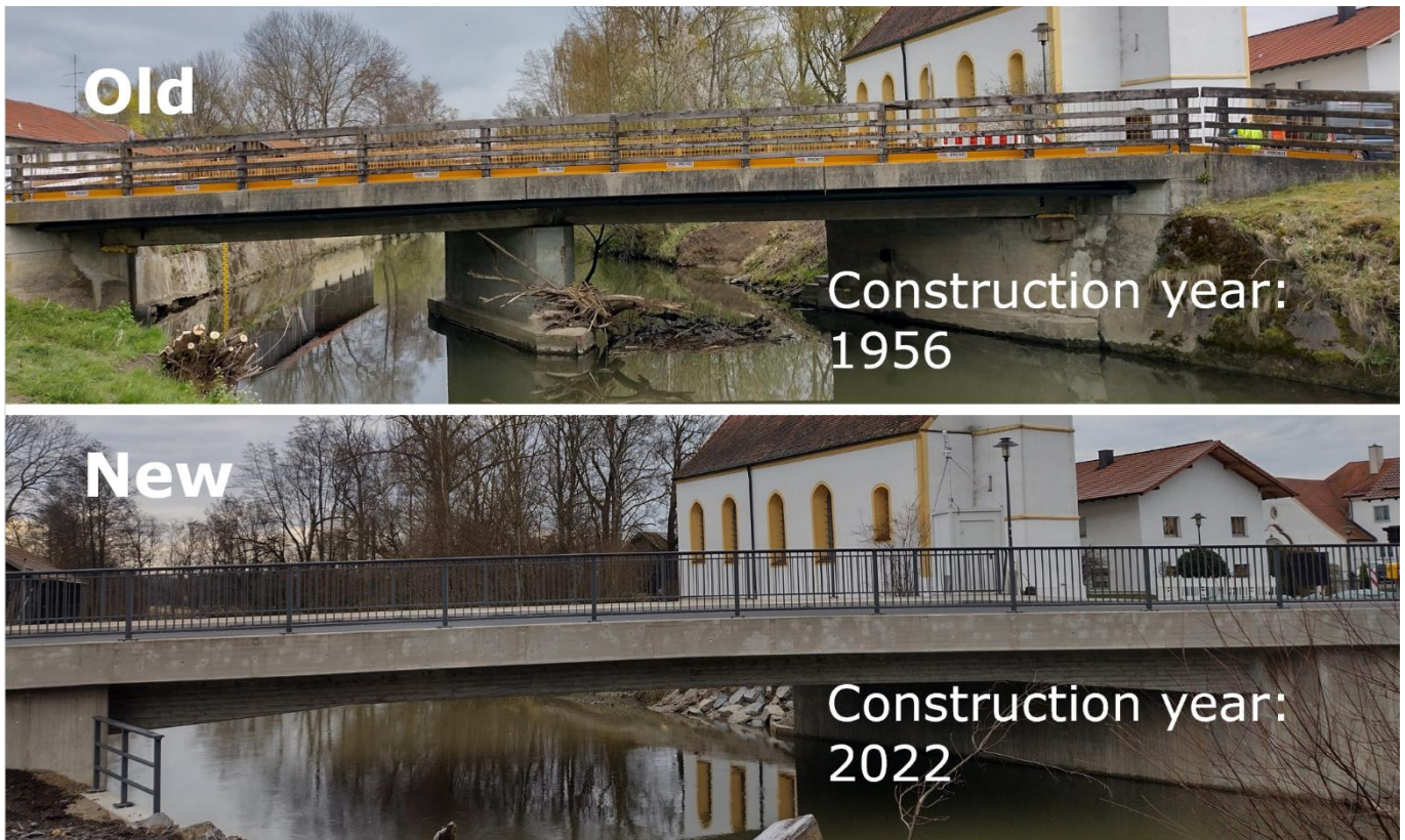
Figure 1 Sideview of the demolished bridge (top) and the new bridge (bottom).
